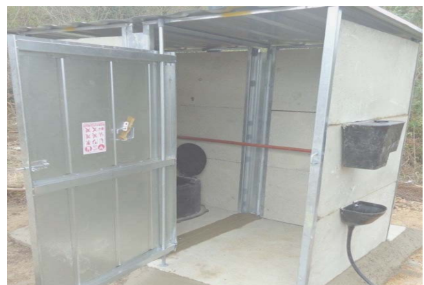
Fig. 4. Improved pit latrine built at an unidentified household in Mpofana
