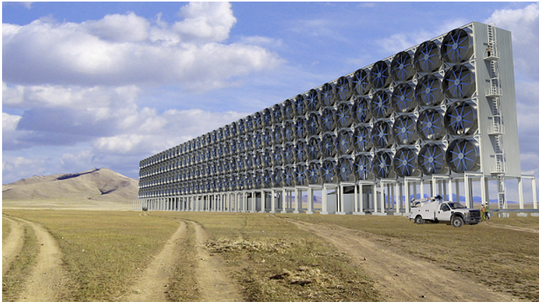
Fig. 3. A rendering of Carbon Engineering's air contactor
